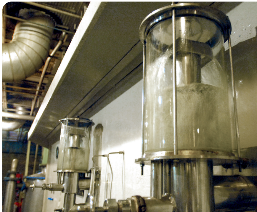
Bioethanol production plant (Courtesy UNICA/ Photo: Niels Andreas)
