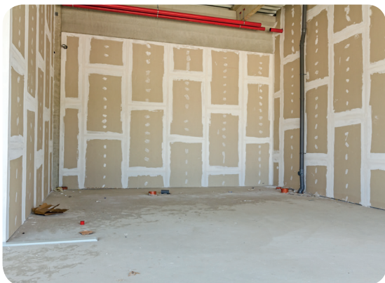
Figure 1: Dry wall panels made of gypsum at building site
