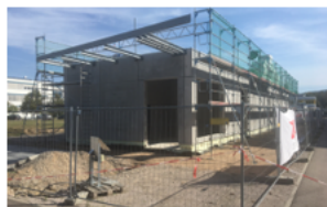
Construction work of the European return hub
